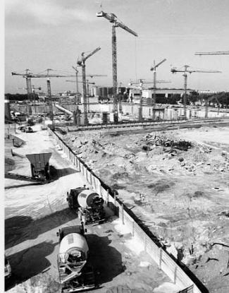
Tall, strong cranes are used to build tall buildings. Cranes lift heavy loads of building material. The cranes are put together near the top of the building. When the building is finished the cranes are taken apart to get them down.
